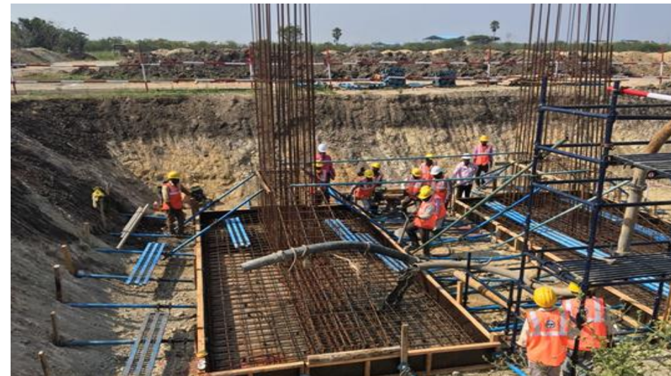
Construction of Tuticorin II (400kt)
