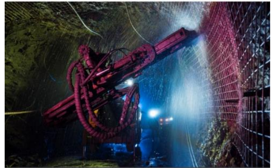
Underground mining operations at Rampura Agucha mine
